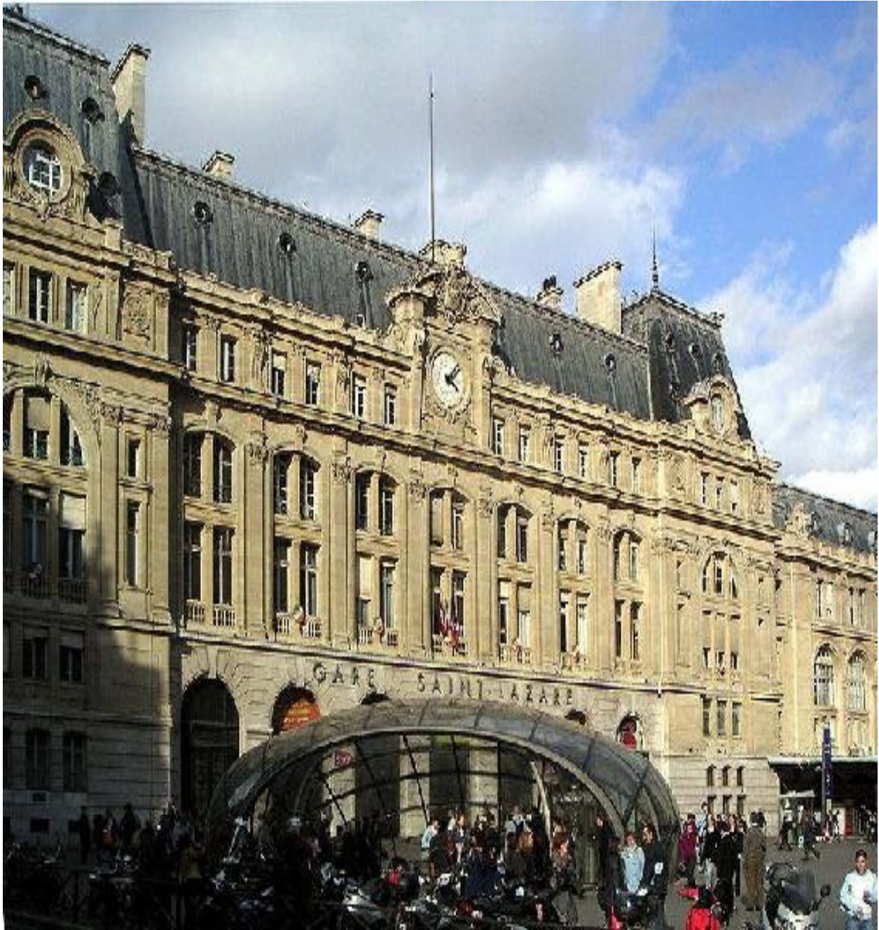
Paris Saint-Lazare, one of the six large terminus train stations of Paris and now immortalised by the artist
