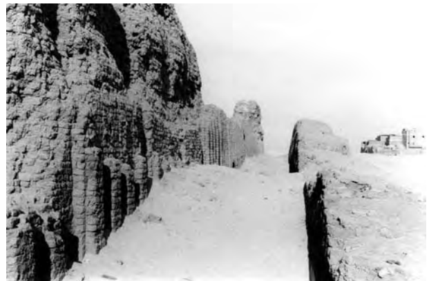
Sun-baked mud brick was the most ancient, and most widely used, building material in ancient Egypt. This is part of the funerary enclosure of Khasekhemwy, the last king of the Second Dynasty, at Abydos, and displays the characteristic paneled motif seen on many monuments of this period. Photo © Aidan Dodson.
