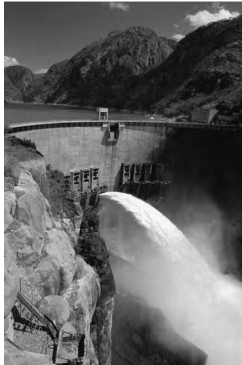
Cabora Bassa Dam, Mozambique. © Friedrich Stark/Das Fotoarchiv.
