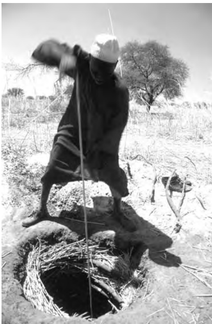
Digging a well, Gredaya, Chad. © Frank Kroenke/Das Fotoarchiv.
