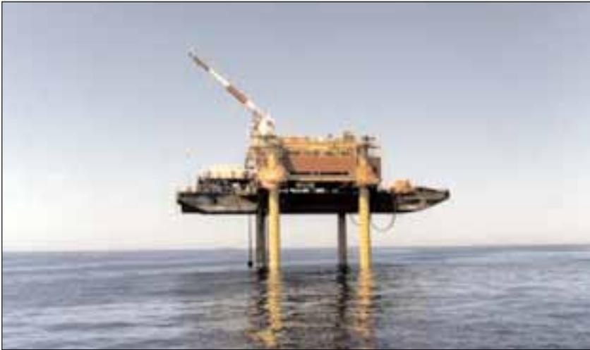
Unocal Q1 Halfweg Platform was installed in March 1995 in the Dutch sector of the southern North Sea. It was designed for “self installation” and consists of a concrete gravity base which supports a manned process deck by means of four tubular steel legs in 24 meters water depth.
