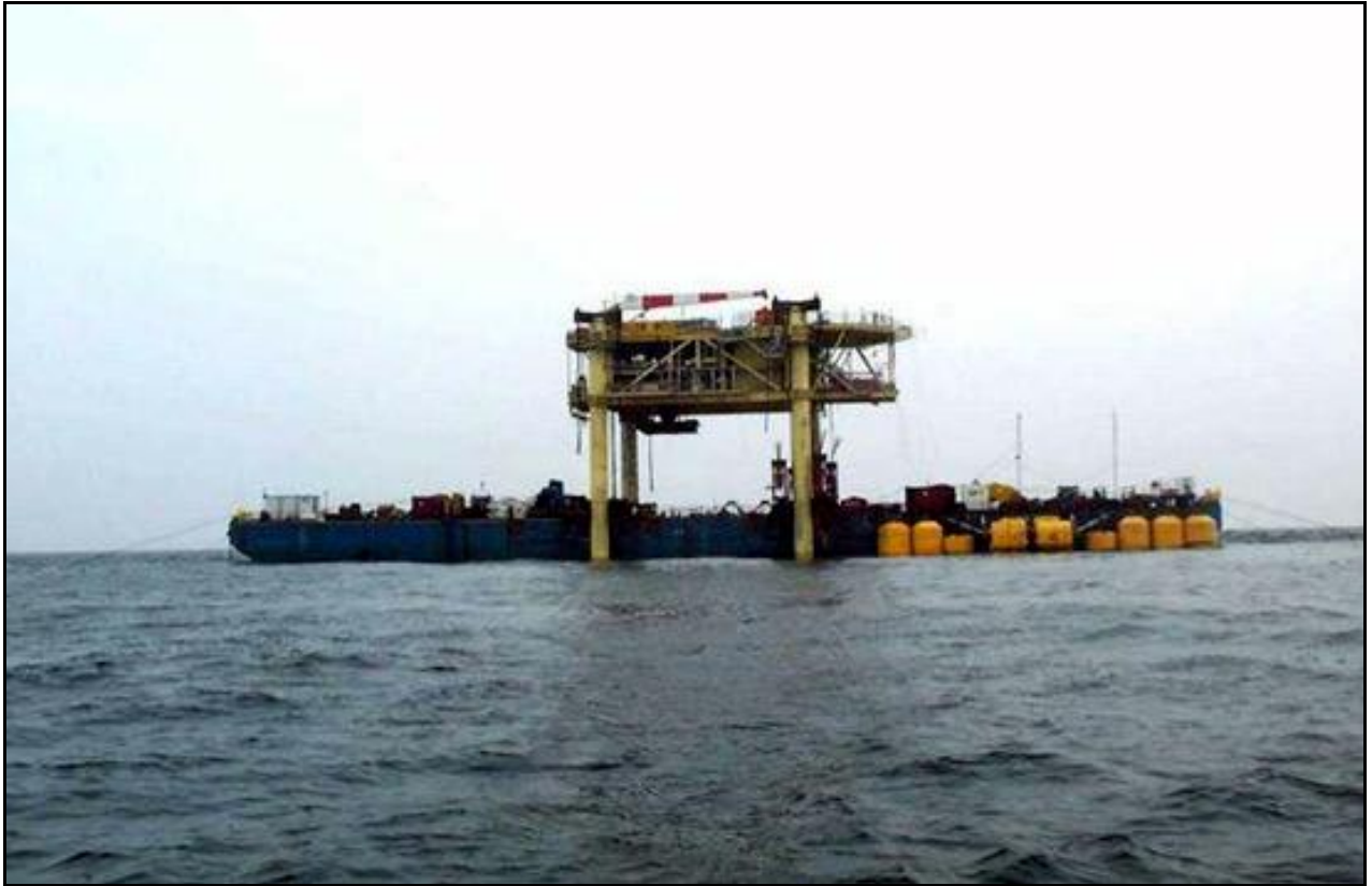
Millom West SeaNode stands in a water depth of 33m but is designed to a capability of 39 metres.
