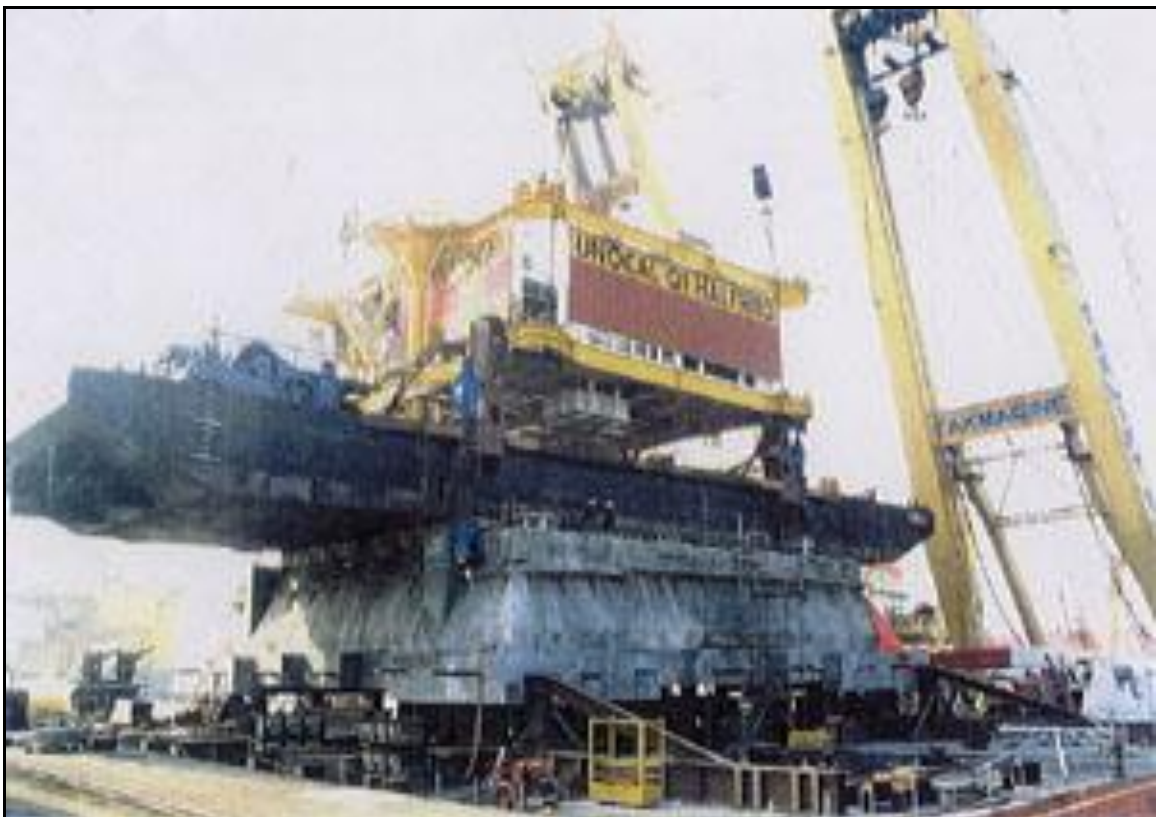
Halfweg Platform in Fabrication yard complete with gravity base, topsides (including integrated Helideck) ready for leg attachment. The topside structure is lowered for transit with the transit/installation barge in position.
