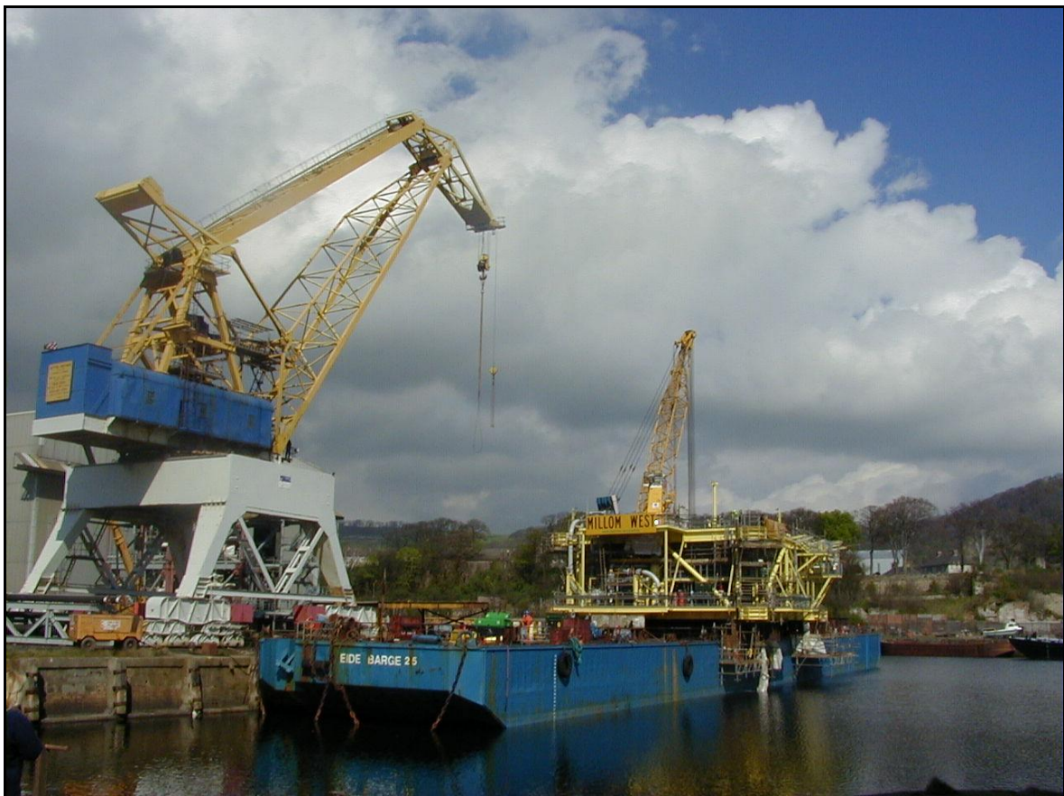
Millom West topside module in the fabrication yard located on transit / installation barge
