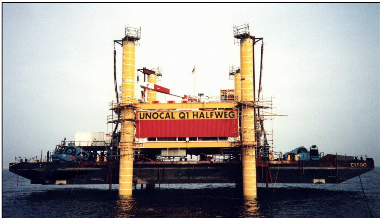
The weight of the barge is used to settle the GBS into the seabed.
